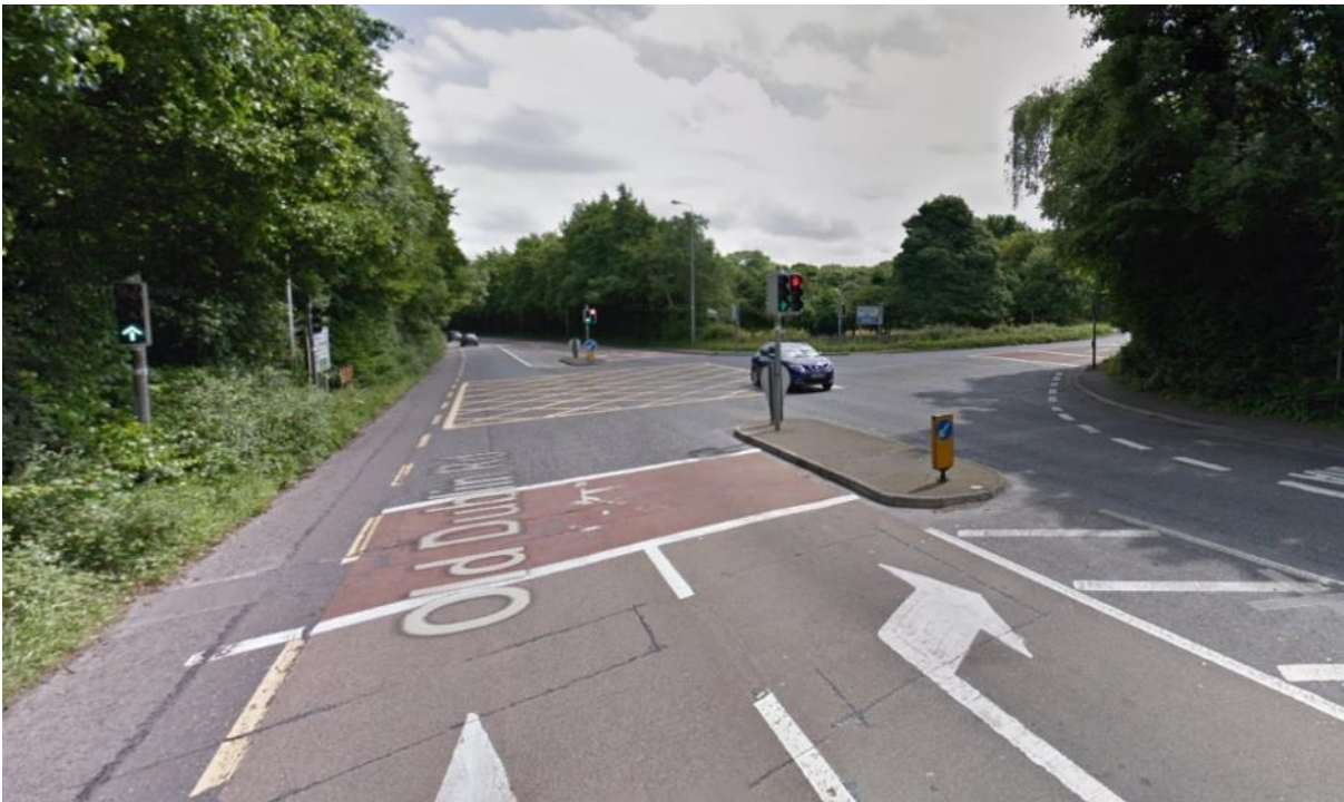
Figure 11.3: Existing Junction (Looking Eastward)
